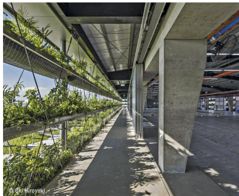
➤ Sliding polycarbonate dividers, fixed in front of the factory's concrete support columns, can be closed in extreme weather.
